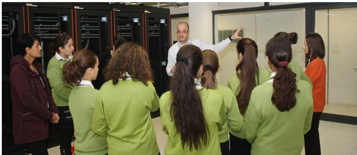
A school visit to the MITA Data Centre.
